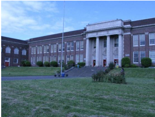
Main building (274A), south (front) and east (side) elevations, looking northwest.
