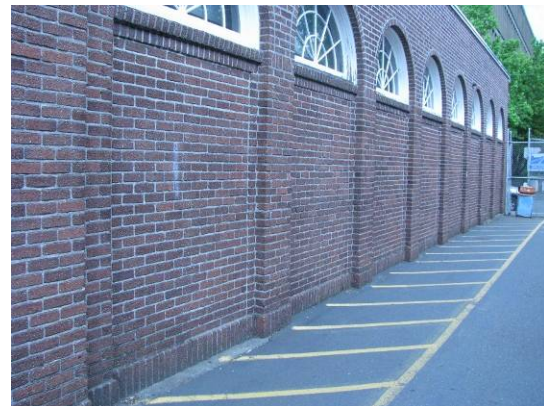
Main building (274A), side entrance along east (side) elevation, looking north.
