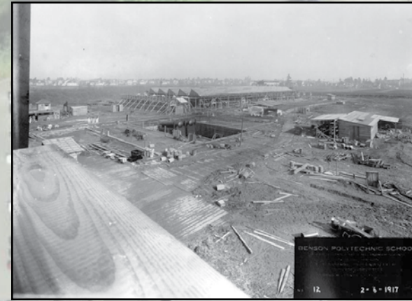
Construction of Benson High School Industrial Arts Building from scaffolding of first unit, looking northeast, 1917.
