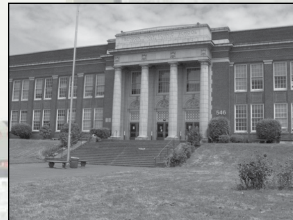
2009 photograph of the front (west) elevation of the Benson High School.
