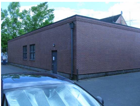
Main building (274A), west (side) elevation, looking northeast.
